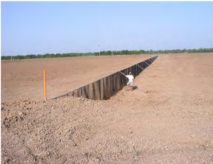
Figure 8. Construction of a commercial-scale confinement system in a 6-ha earthen pond in Chicot County, Arkansas.
